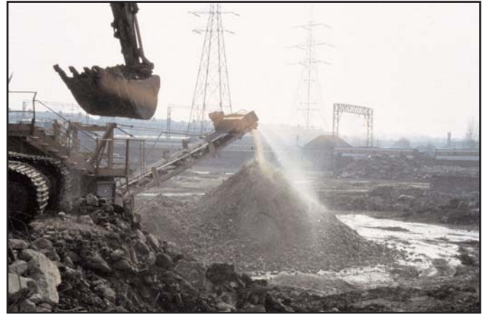
Soil sorting and crushing- a physical treatment
