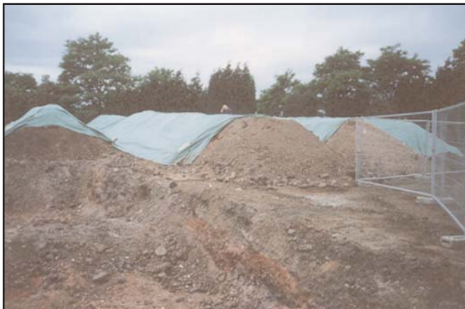
Biopiling- Biological treatment of soil for organics
